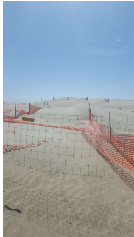
Exhibit 3. 2018 wind fencing projects installed at Oceano Dunes SVRA. Partially buried fencing requiring maintenance is visible in the top and lower right photographs.
