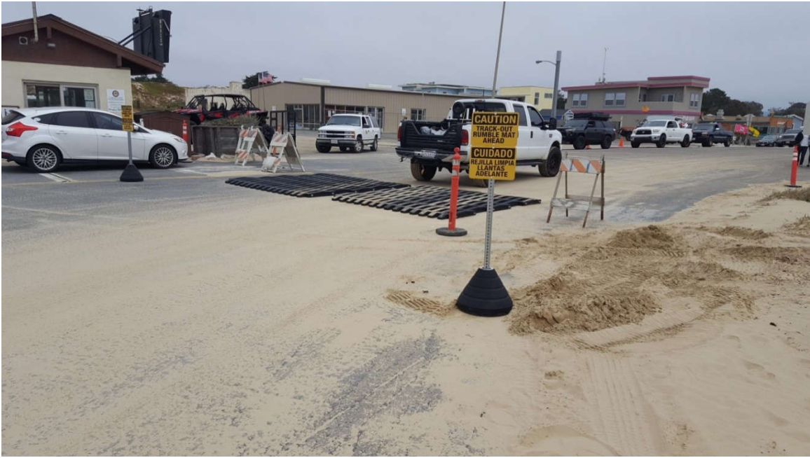
Exhibit 4. Pier Avenue Trackout Mats.
