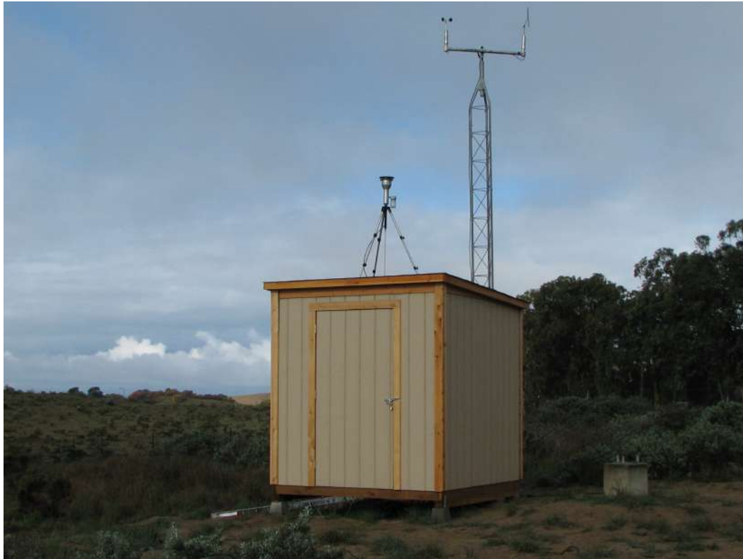
Figure 3.12 – CDF Monitoring Station (Northwest View)
