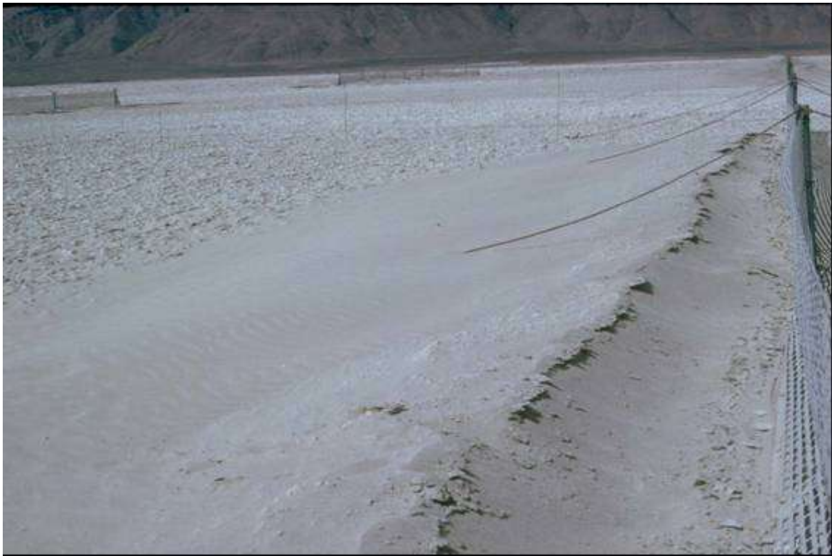
Figure C 81 - Detail of partially built sand dune
