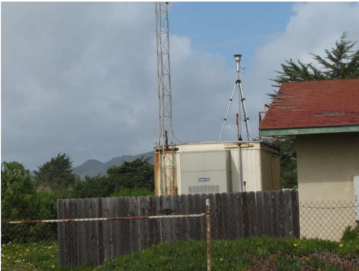
Figure 3.2 - Grover Beach Monitoring Station (North View)
