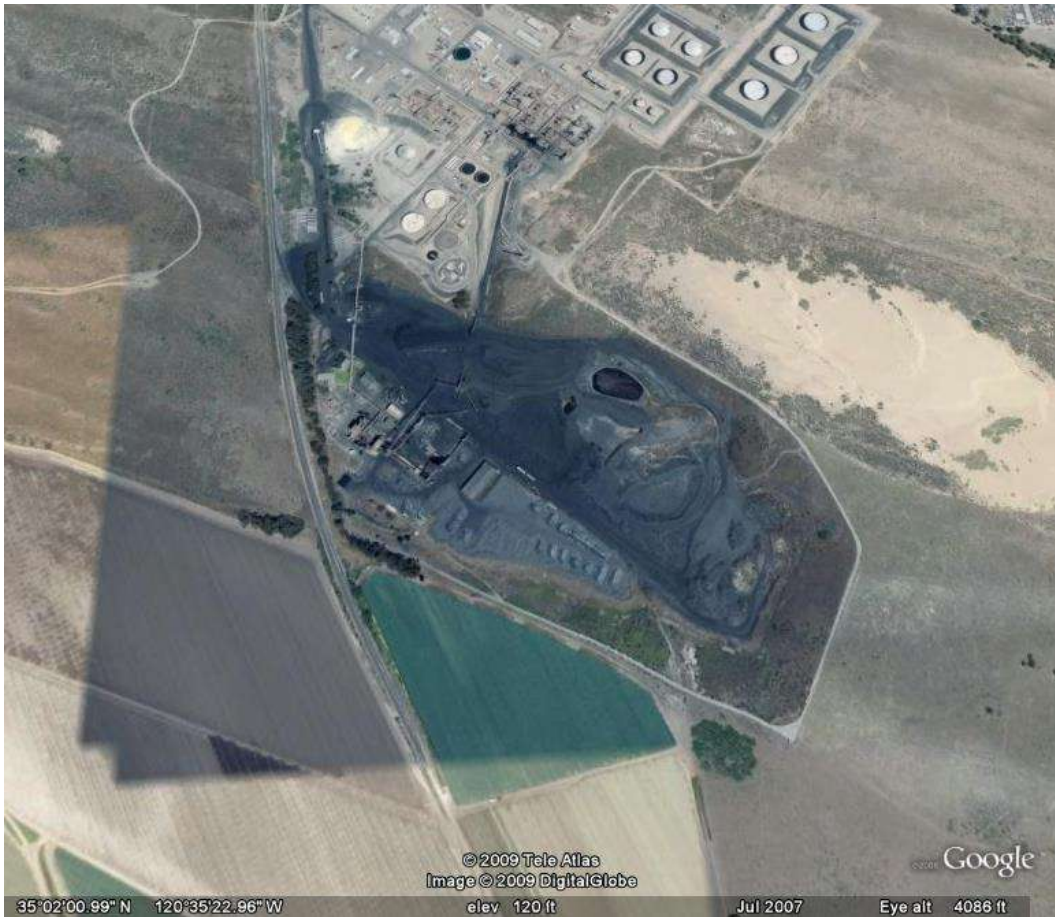
Figure C 54 - The ConocoPhillips refinery and coke pile - The ConocoPhillips refinery and coke pile
