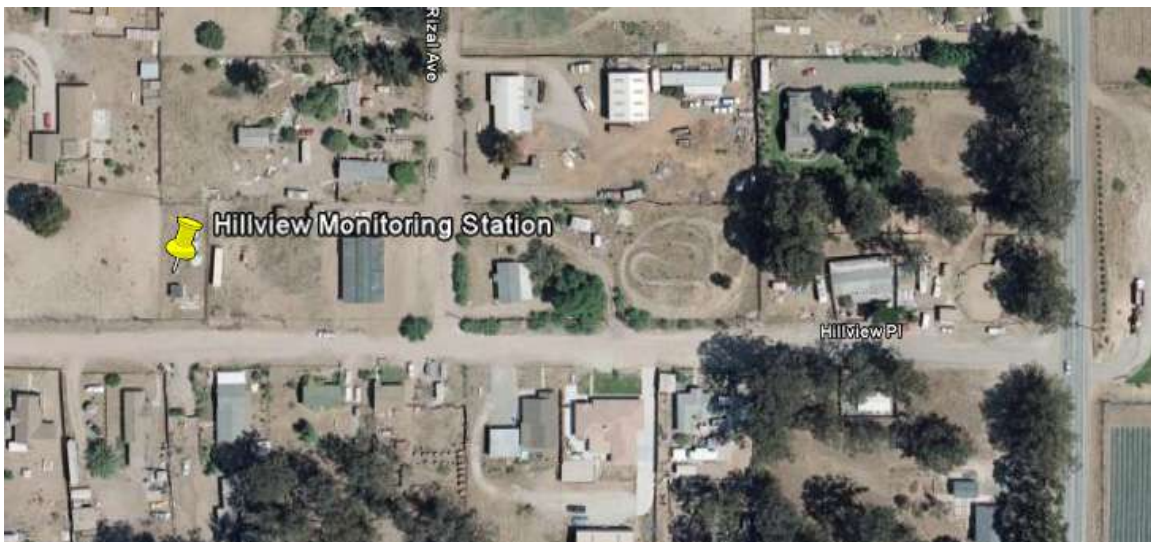
Figure 3.17 - Aerial View of Hillview Monitoring Station
