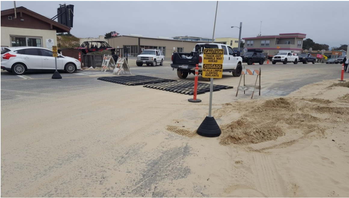
Exhibit 4. Pier Avenue Trackout Mats.
