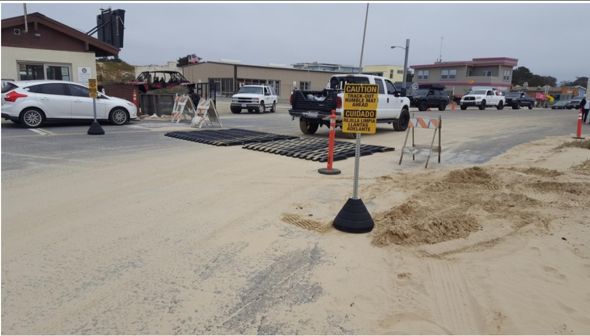
Exhibit 4. Pier Avenue Trackout Mats.
