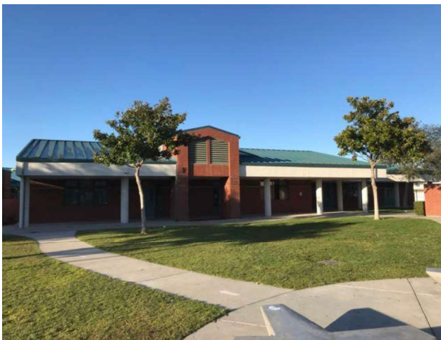
5 - EXTERIOR ELEVATION, BUILDING F
