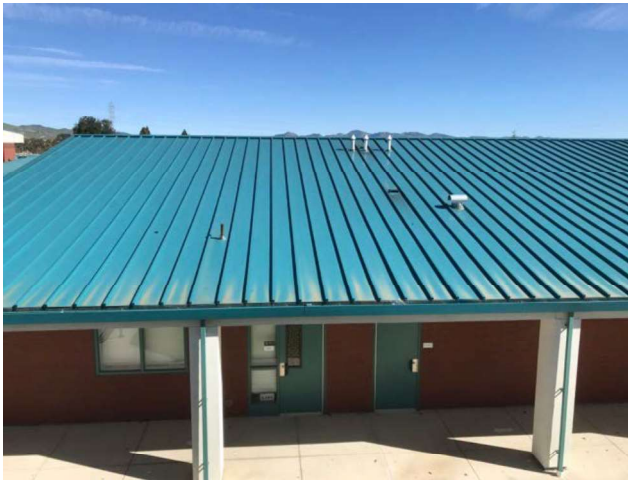
9 - METAL ROOFING OVERVIEW
