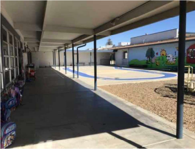
19 - COVERED WALKWAY, KINDERGARTEN
