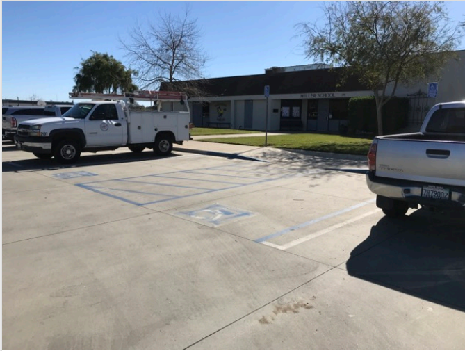
Overview of accessible parking area
