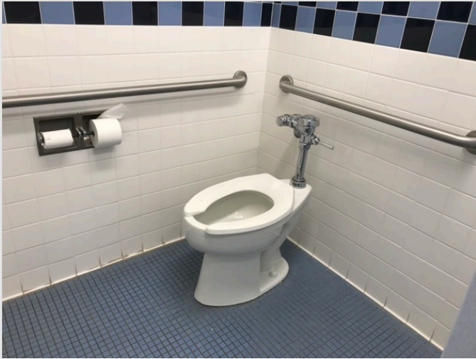
Toilet stall overview
