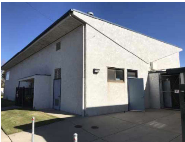
11 - LEFT ELEVATION, CAFETERIA
