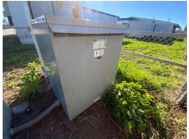
28 - SECONDARY TRANSFORMER
