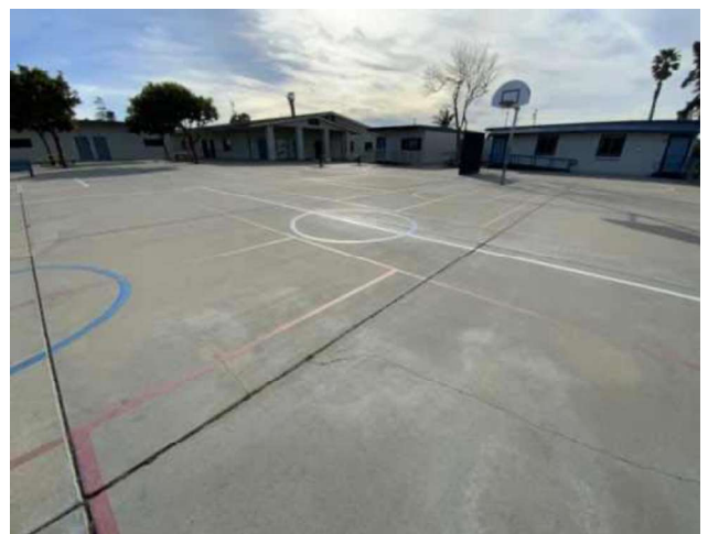
36 - CONCRETE SPORTS COURTS
