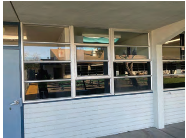
8 – WINDOWS, DOORS, AND FACADE
