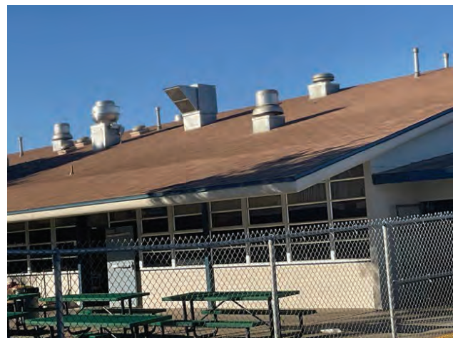
6 – ASPHALT SHINGLES ROOFING
