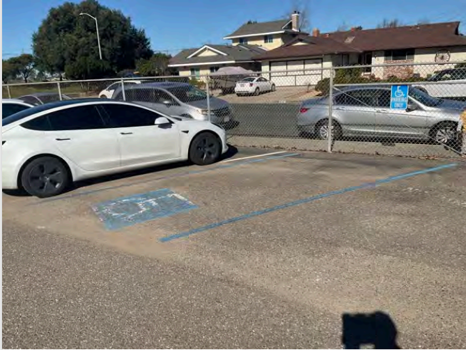
OVERVIEW OF ACCESSIBLE PARKING AREA
