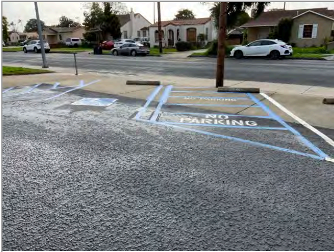
OVERVIEW OF ACCESSIBLE PARKING AREA
