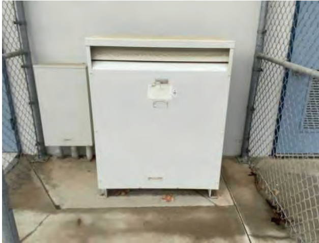
25 - SECONDARY TRANSFORMER
