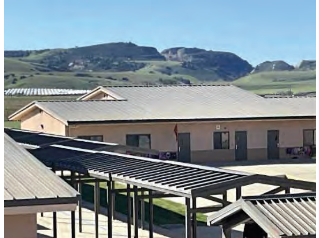
8 - SECONDARY ROOF OVERVIEW
