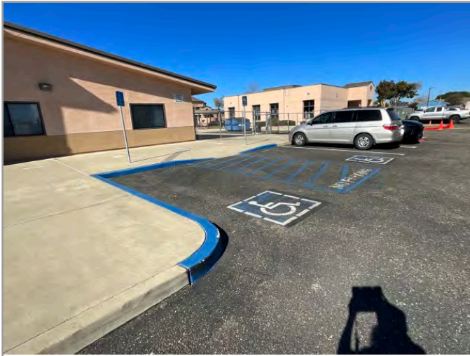
OVERVIEW OF ACCESSIBLE PARKING AREA
