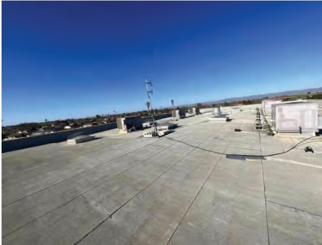
7 - PRIMARY ROOF OVERVIEW
