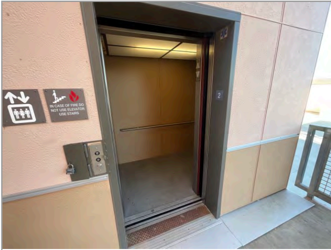
LOBBY LOOKING AT CABS (WITH DOORS OPEN)
