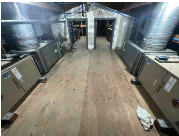
17 - ATTIC FURNACE SPACE
