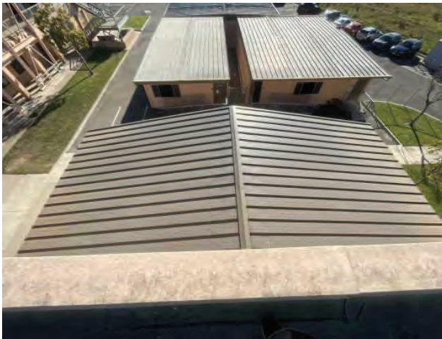
9 - SECONDARY ROOF OVERVIEW
