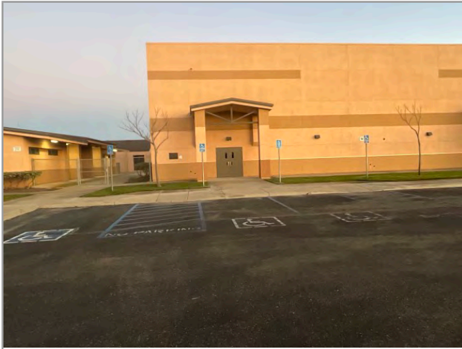
OVERVIEW OF ACCESSIBLE PARKING AREA
