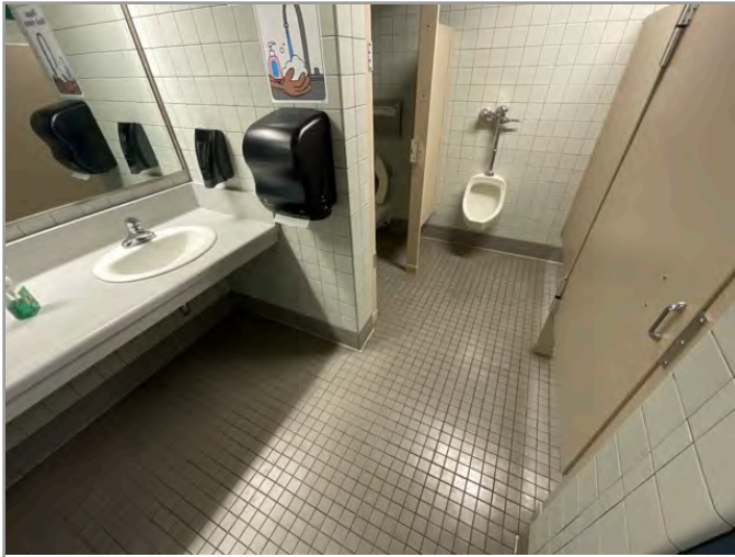
TOILET STALL OVERVIEW
