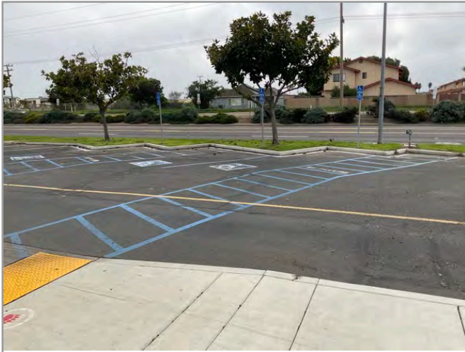
OVERVIEW OF ACCESSIBLE PARKING AREA
