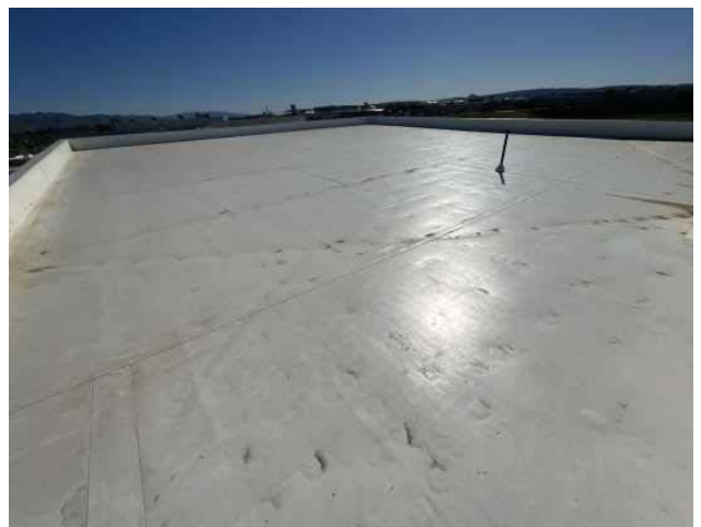
6 - PRIMARY ROOF OVERVIEW
