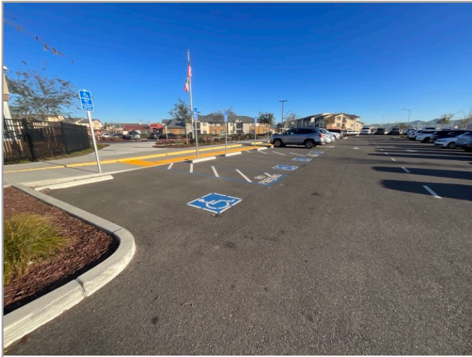
OVERVIEW OF ACCESSIBLE PARKING AREA
