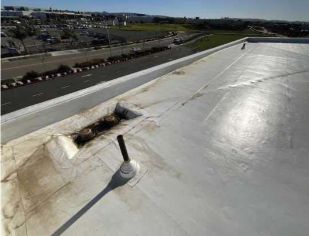
7 - DRAINAGE / PARAPET WALL
