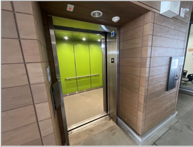
LOBBY LOOKING AT CABS (WITH DOORS OPEN)
