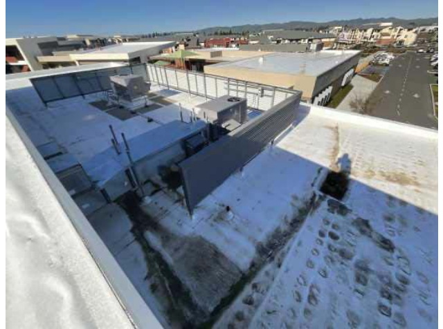
8 - SECONDARY ROOF OVERVIEW
