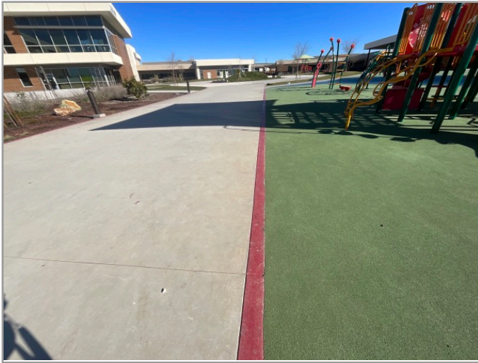
ACCESSIBLE ROUTE TO PLAYGROUND
