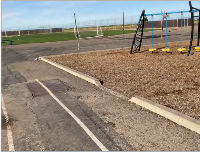
ACCESSIBLE ROUTE TO PLAYGROUND
