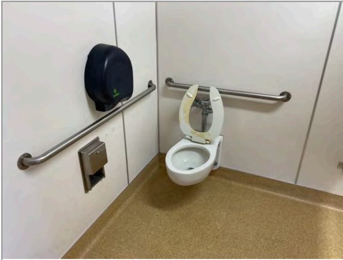
TOILET STALL OVERVIEW
