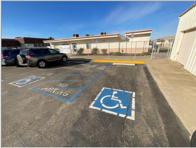
OVERVIEW OF ACCESSIBLE PARKING AREA
