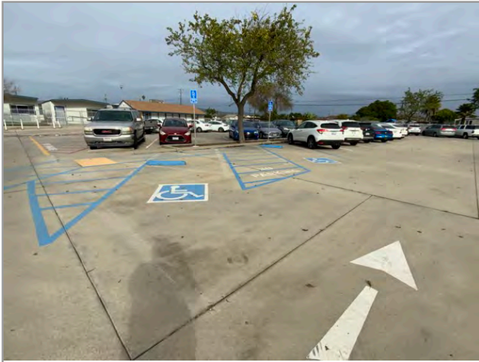
OVERVIEW OF ACCESSIBLE PARKING AREA
