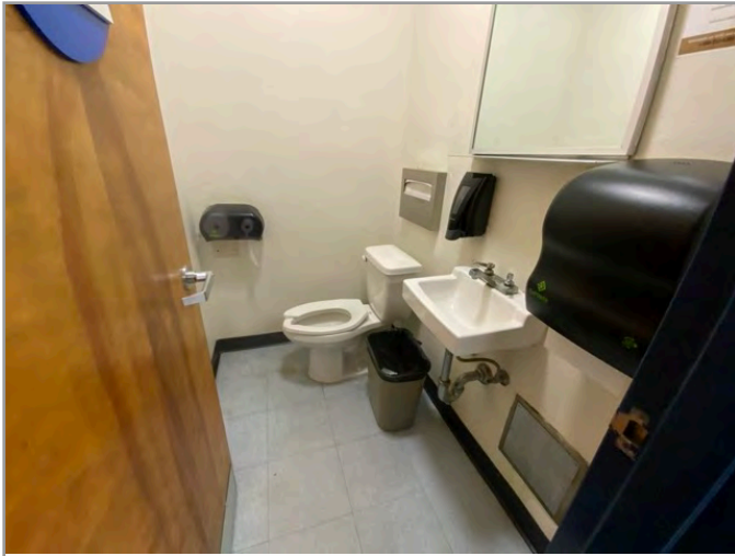
TOILET STALL OVERVIEW
