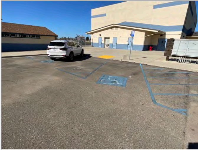
OVERVIEW OF ACCESSIBLE PARKING AREA
