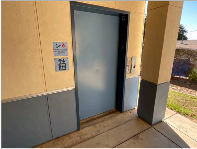
LOBBY LOOKING AT CABS (WITH DOORS OPEN)
