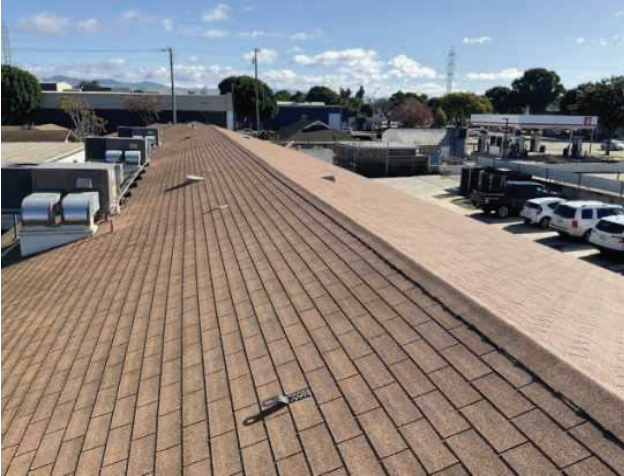
7 - ASPHALT SHINGLE ROOFING
