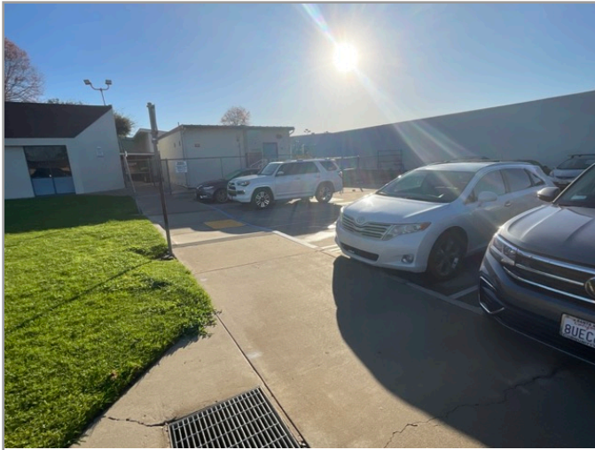
OVERVIEW OF ACCESSIBLE PARKING AREA
