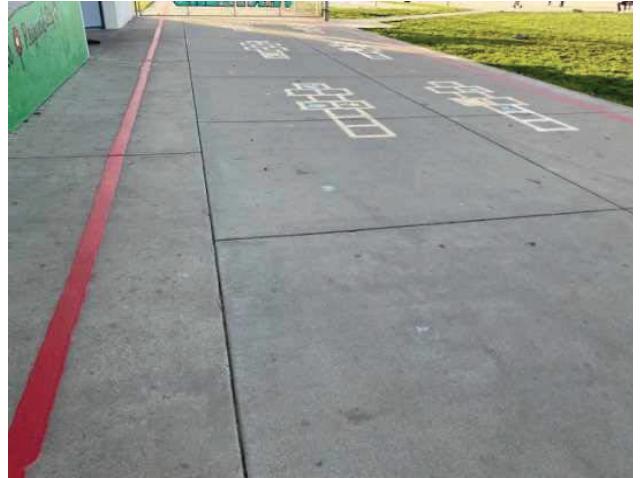
32 - CONCRETE SURFACES THROUGHOUT
