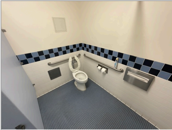
TOILET STALL OVERVIEW
