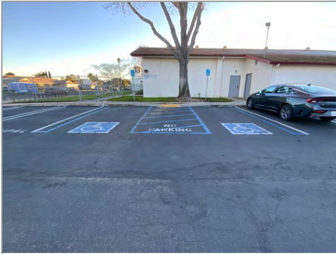
OVERVIEW OF ACCESSIBLE PARKING AREA
