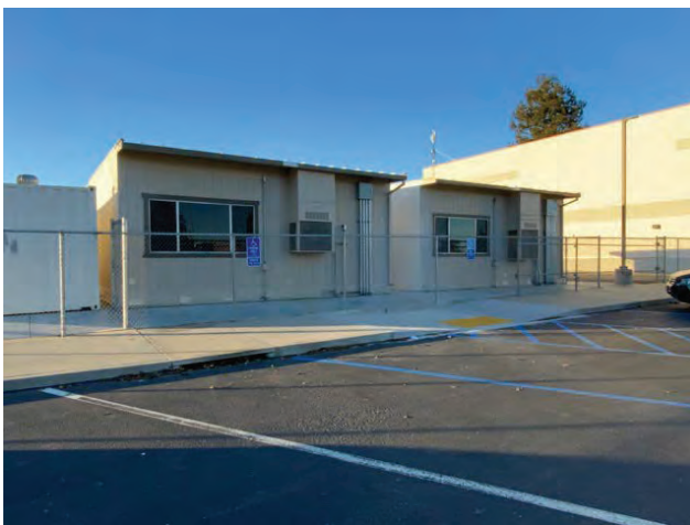
47 - ACCESSIBLE PARKING AREA
