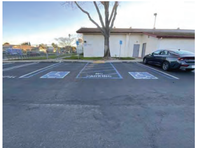
46 - ACCESSIBLE PARKING AREA
