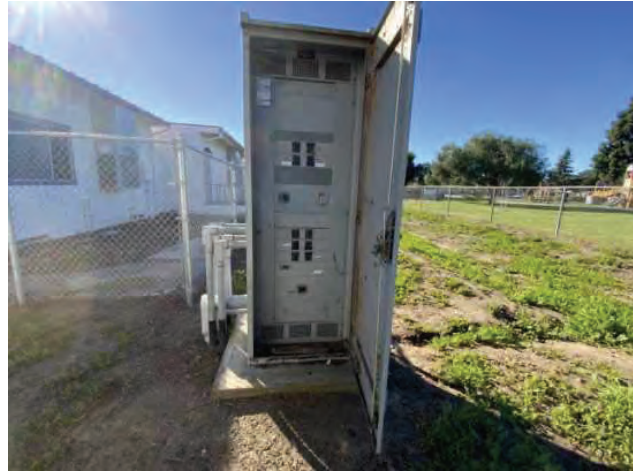
32 – ELECTRICAL SWITCHBOARD
