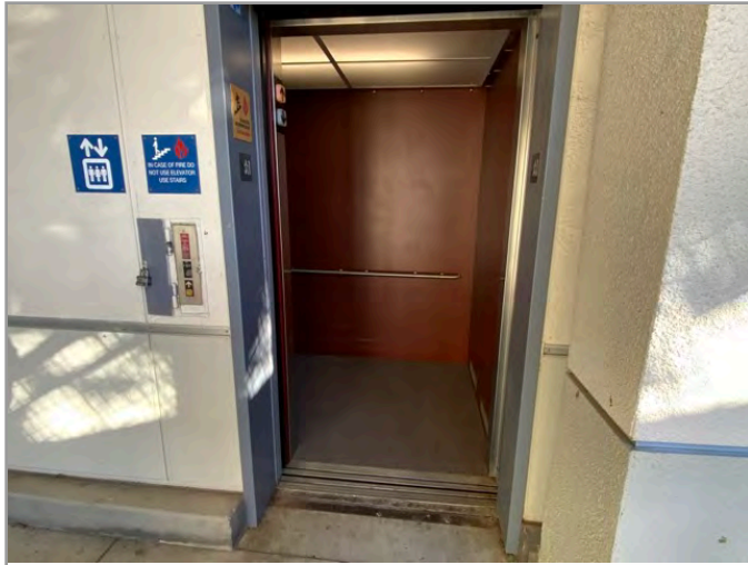
LOBBY LOOKING AT CABS (WITH DOORS OPEN)
