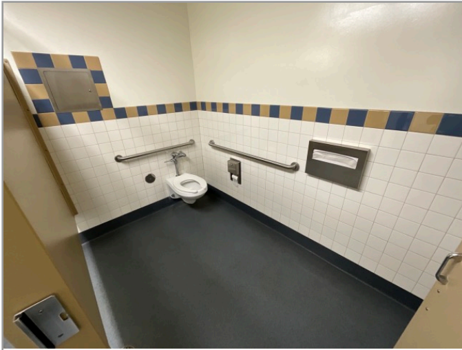
TOILET STALL OVERVIEW
