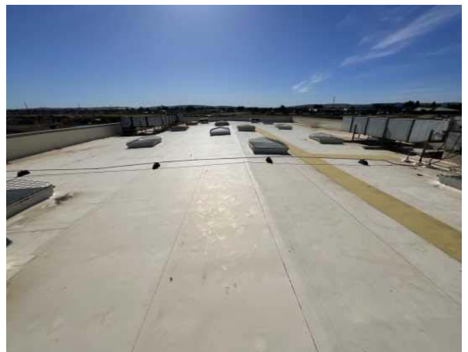
6 - PRIMARY ROOF OVERVIEW
