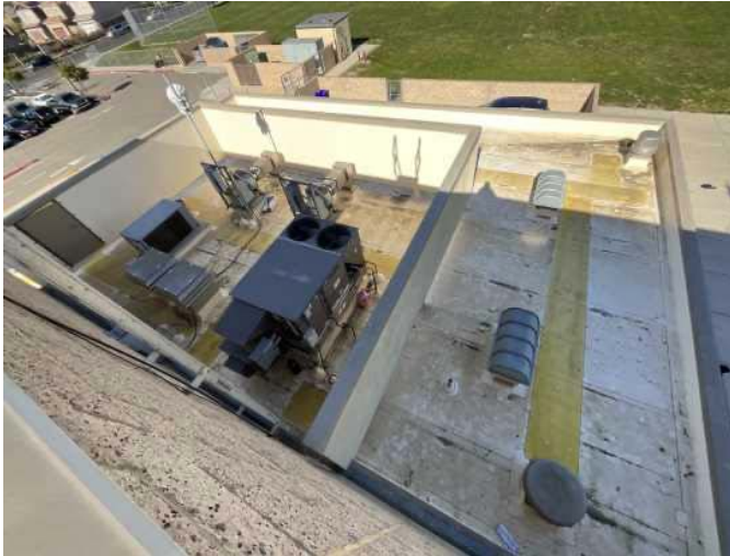
19 - SECONDARY ROOF OVERVIEW
