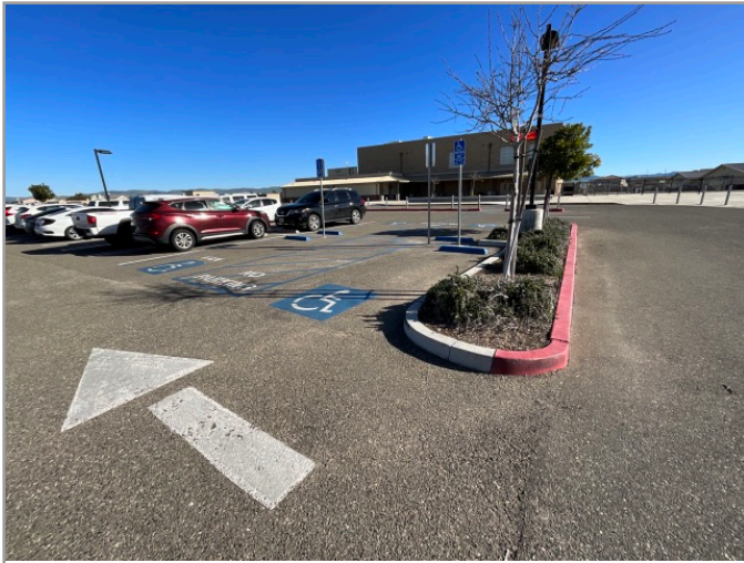
OVERVIEW OF ACCESSIBLE PARKING AREA
