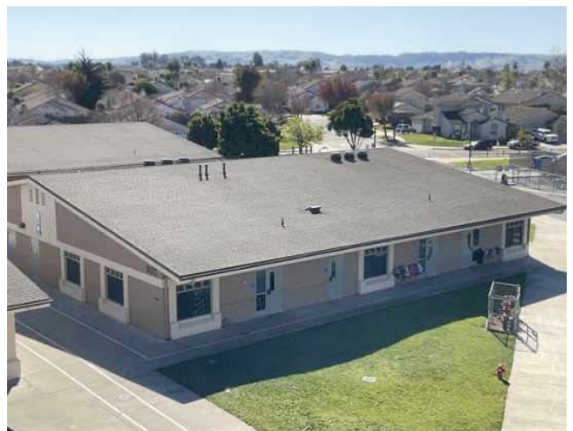
6 - ASPHALT SHINGLE ROOFING
