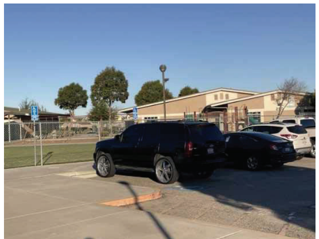
36 - OVERVIEW OF ACCESSIBLE PARKING AREA
