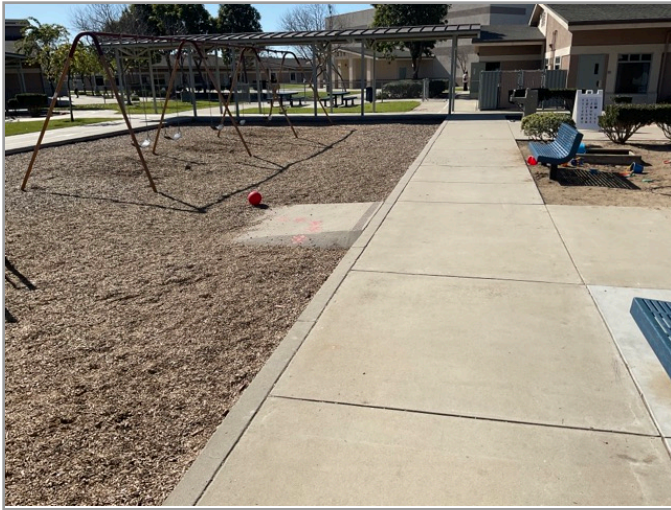
ACCESSIBLE ROUTE TO PLAYGROUND
