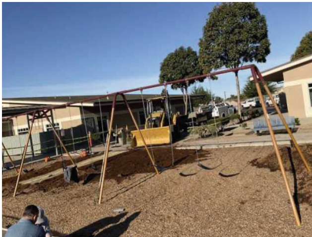
33 - INSTALLATION OF NEW RAMP
