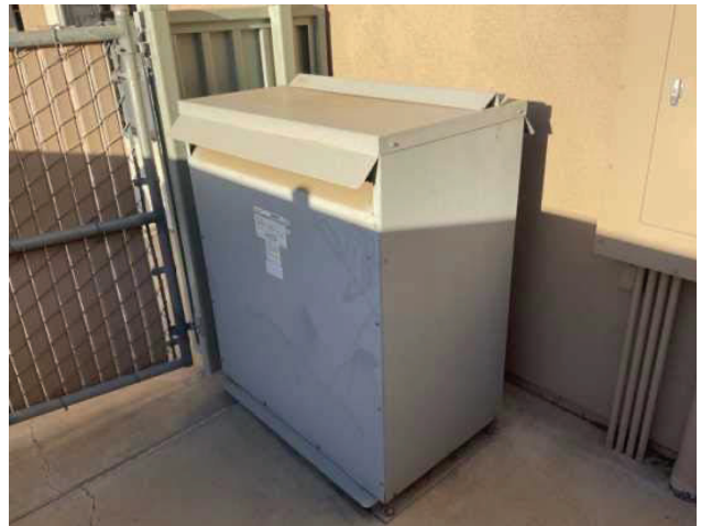
22 - SECONDARY TRANSFORMER
