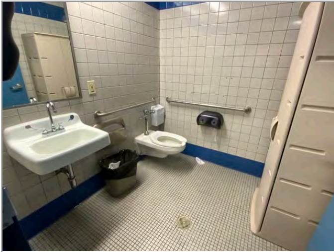
TOILET STALL OVERVIEW
