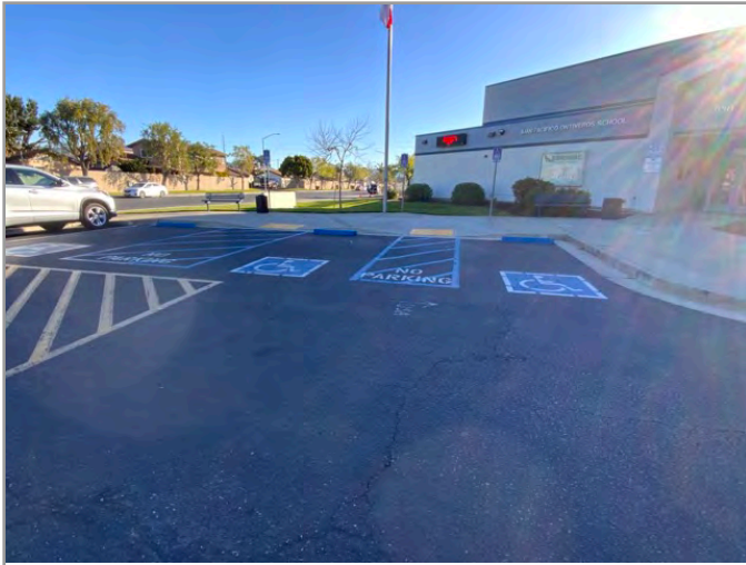
OVERVIEW OF ACCESSIBLE PARKING AREA
