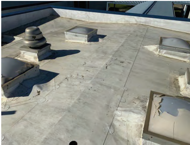
13 - DAMAGED SKYLIGHTS
