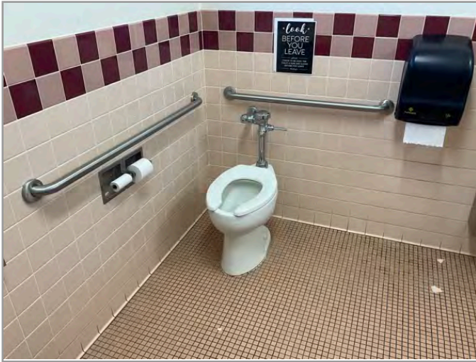
TOILET STALL OVERVIEW
