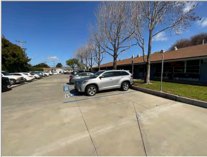
OVERVIEW OF ACCESSIBLE PARKING AREA
