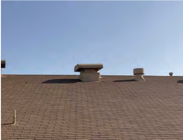
7 - ASPHALT SHINGLE ROOF
