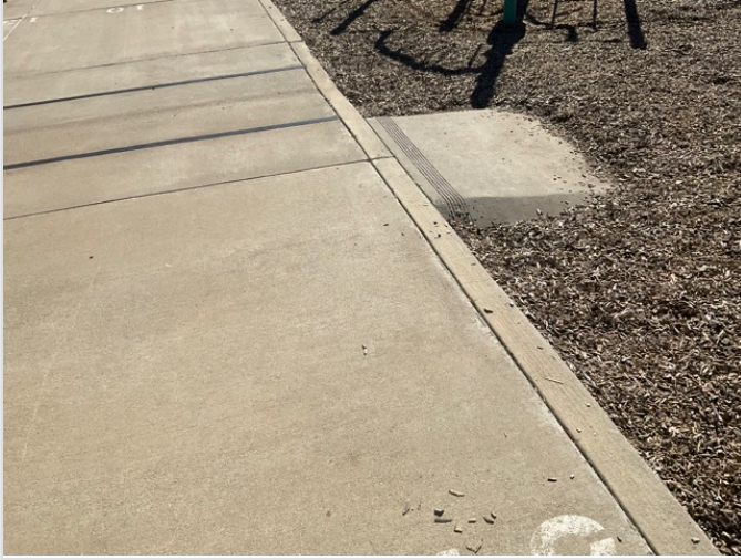
ACCESSIBLE ROUTE TO PLAYGROUND
