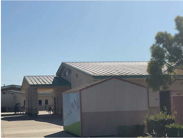
7 – METAL FINISH ROOFING
