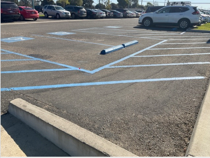
OVERVIEW OF ACCESSIBLE PARKING AREA
