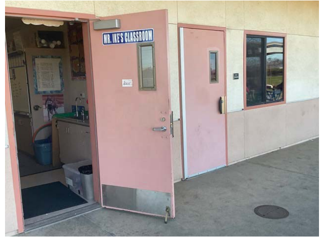
8 – WINDOWS, DOORS, AND FACADE
