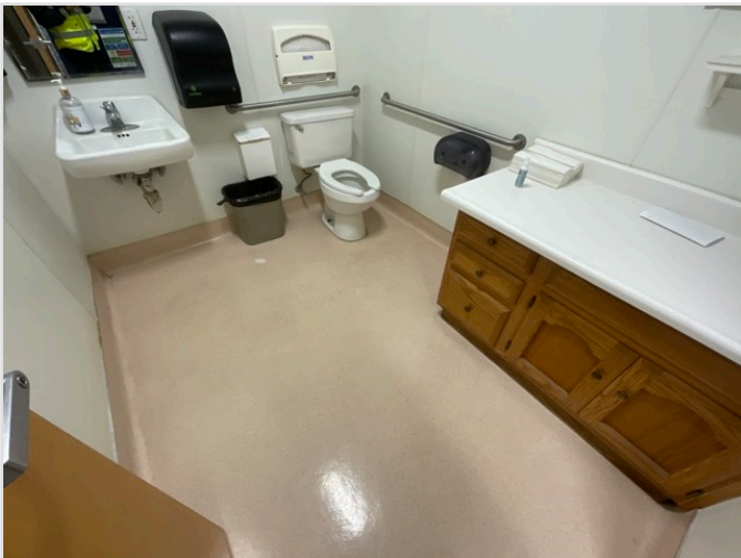
TOILET STALL OVERVIEW
