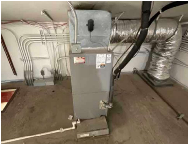
21 - SPLIT SYSTEM FAN COIL
