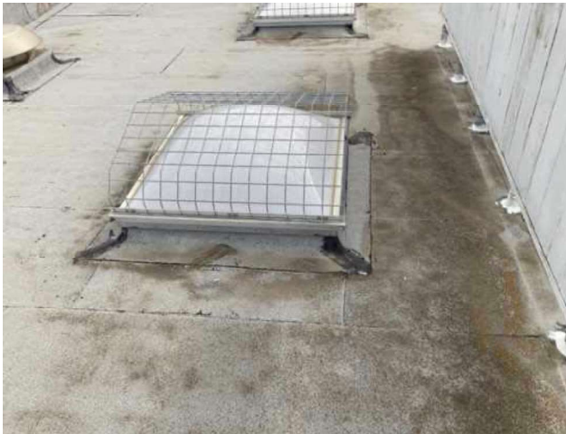
9 - PROTECTED ROOF SKYLIGHT
