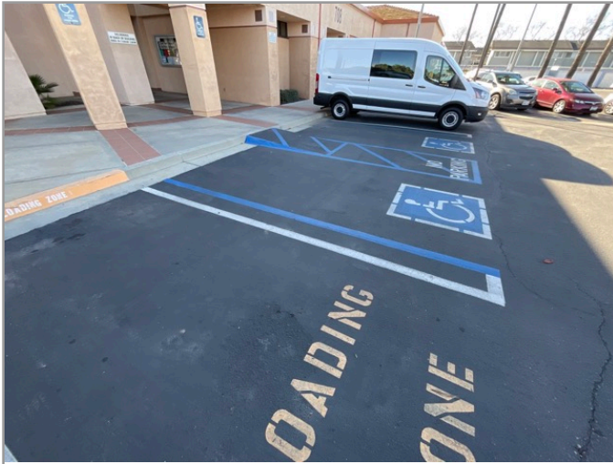
OVERVIEW OF ACCESSIBLE PARKING AREA
