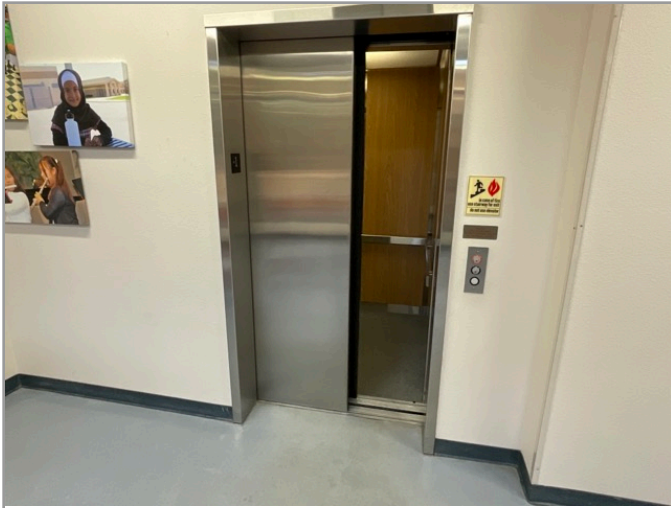
LOBBY LOOKING AT CABS (WITH DOORS OPEN)
