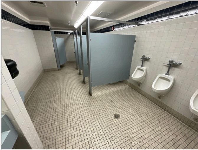
TOILET STALL OVERVIEW
