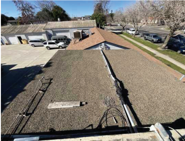
7 - SECONDARY ROOF OVERVIEW
