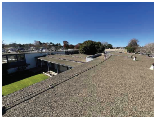
6 - PRIMARY ROOF OVERVIEW
