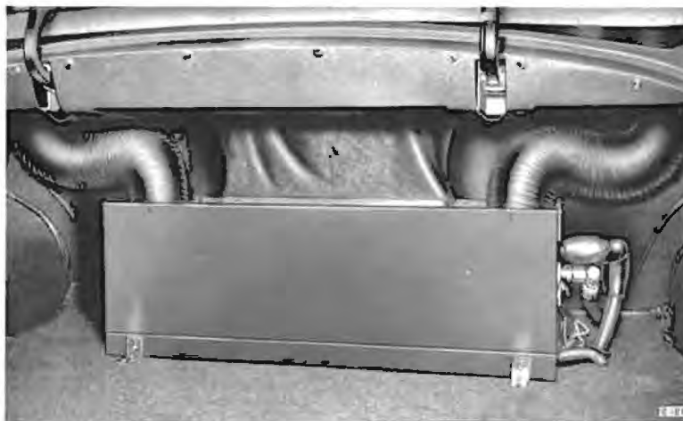
Fig. 3 Evaporator Unit Installed in Boot
