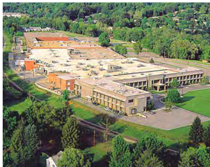
AERUS MANUFACTURING PLANT | BRISTOL, VA
