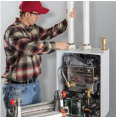
1/2" gas connections (subject to local code) and 2" PVC venting help reduce installation time.
