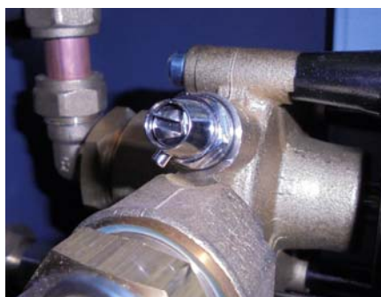
Figure 15 - Priming Screw
