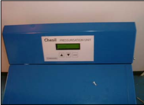
Figure 27 - Display PCB Location Floor Standing Unit
