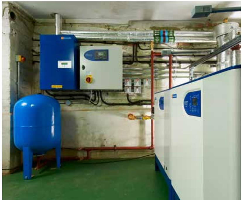
Typical plant room with a wall-mounted Chesil pressurisation unit, Burstock expansion vessel, and Merley sequence controller, supporting an array of Hamworthy Fleet boilers
