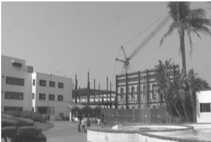
New San Quentin Hospital construction built to accommodate original 1885 facade
