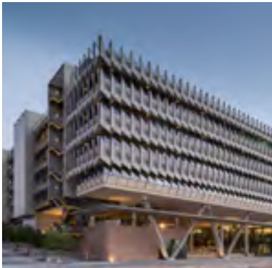
Siemens Middle East HQ
