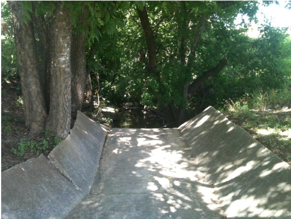
Figure 8-18 Photo of Existing Flume Looking Downstream
