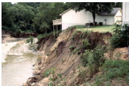
Figure 6-7 Creek Erosion Threatening Home
