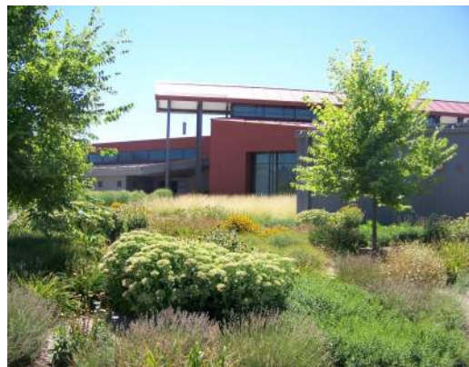
San Pedro Senior High School, Olguin Campus. Photo By: CO Architects
