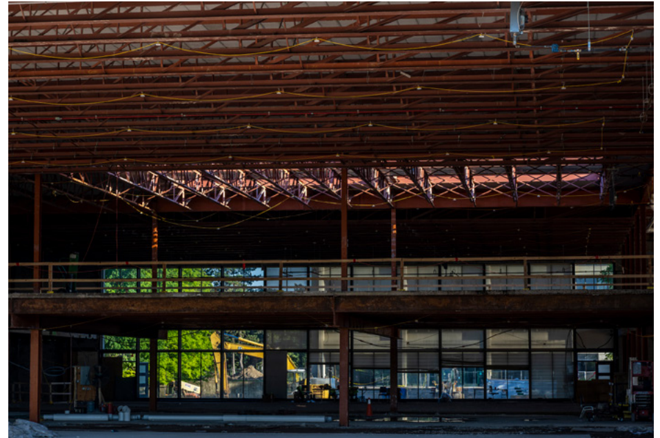
Rehab Hewitt Hall - Phase I
