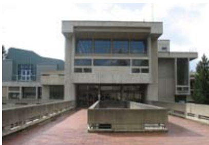
Figure 2.5. The pedestrian bridge connection between CAB and CRC is dysfunctional and disorienting.
