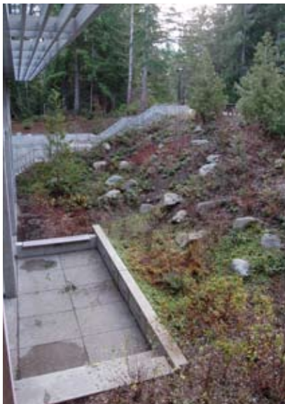
Figure 2.6. Green roofs and bioswales harvest rainwater at SEM II.
