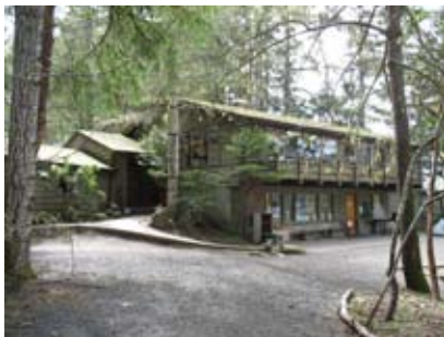
Figure 6.7. Existing Geoduck House
