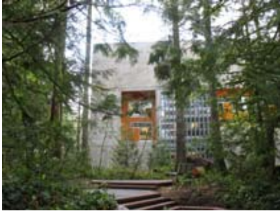
Figure 7.1. Seminar II is integrated into the landscaping which softens and complements the buildings material choices.
