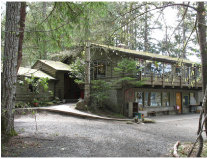
Figure 6.7. Existing Geoduck House
