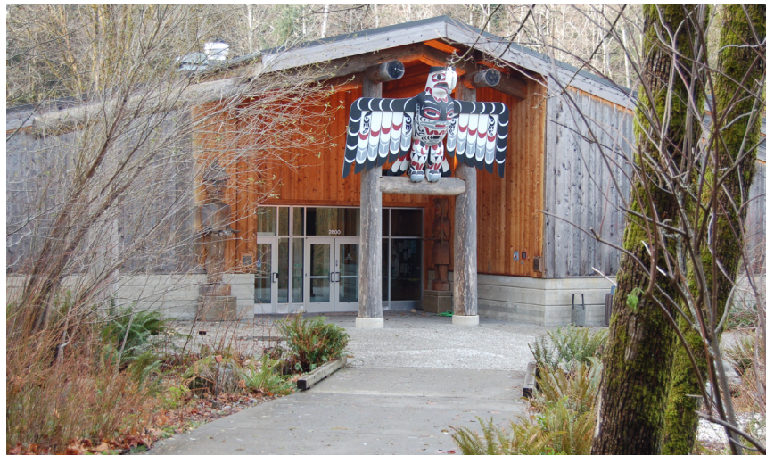
Figure 6.13. The Longhouse and the adjacent ethno-cultural garden are campus landmarks and focal points for Reservation-based programs.
