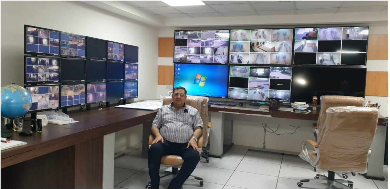
Figure 13: Picture showing the Building Monitoring System while it is functioning
