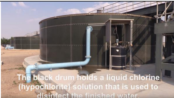
Disinfection and storage facilities of University City Wastewater Treatment Plant
