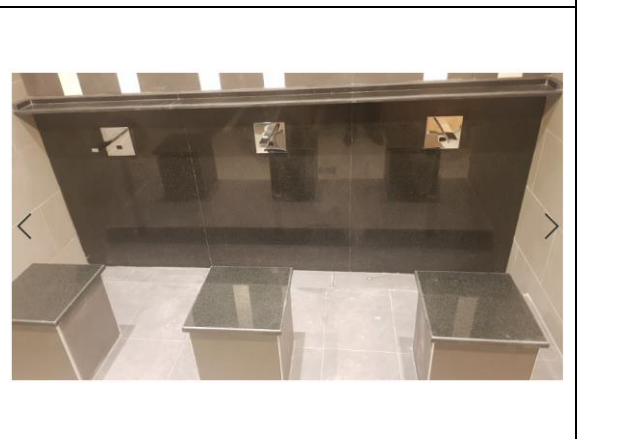
Example of efficient water faucet (low flow type) in ablution area (Photo source: University of Sharjah )
