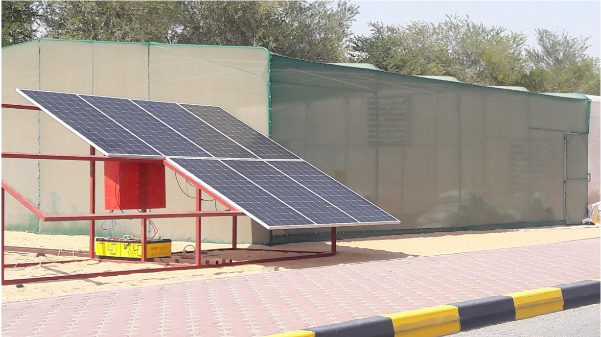
Figure 24: Solar PV (2.52 Kw) Powered Green House – University of Sharjah
