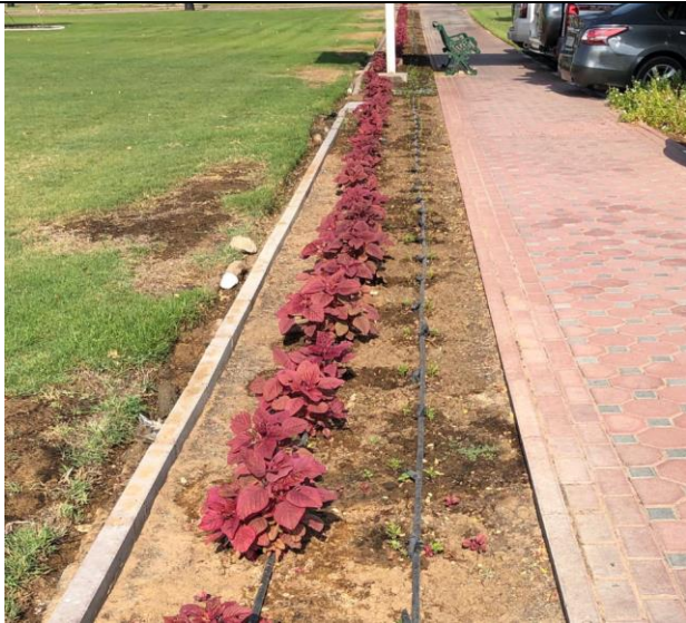
Examples of efficient drip irrigation network (Photo source: University of Sharjah). Plants and flowers in the University are irrigated with a vast drip irrigation system.
