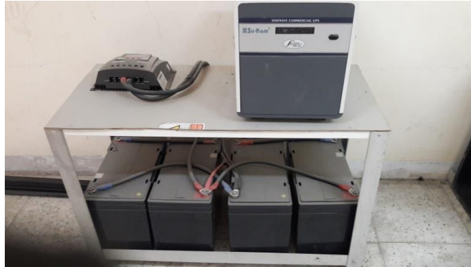
Figure 22: Batteries and Controller, Solar PV for Golf Cart Charging (1.5 kW)
