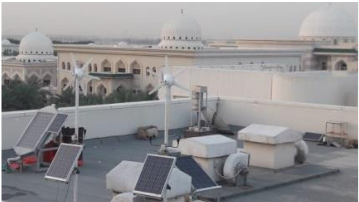
Figure 25: Hybrid Solar PV/Wind Energy system (800 W)
