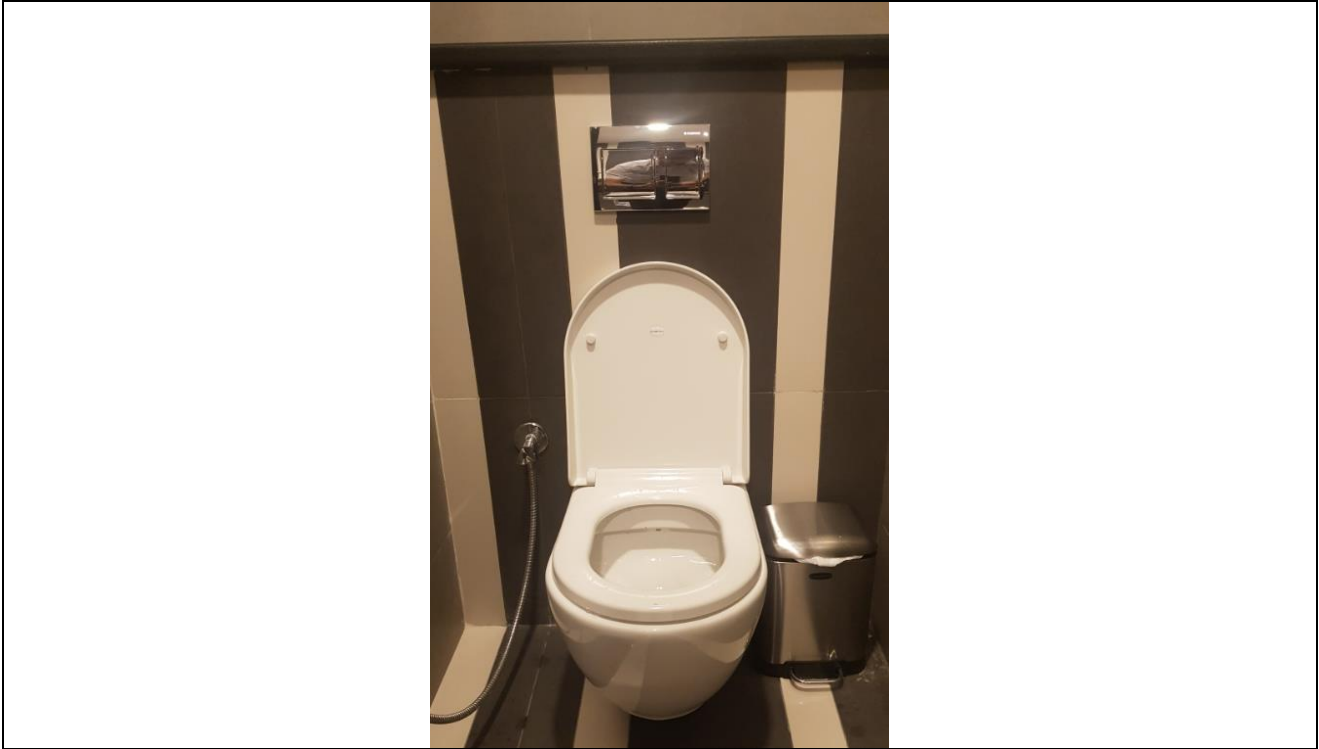
Example of the dual flush low flow toilet (Photo source: University of Sharjah )
