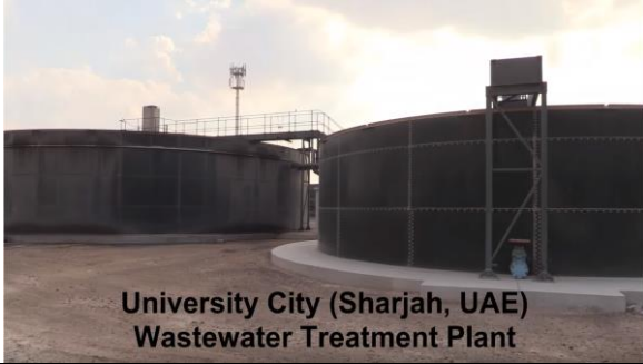
Views of primary clarifier of University City Wastewater Treatment Plant
