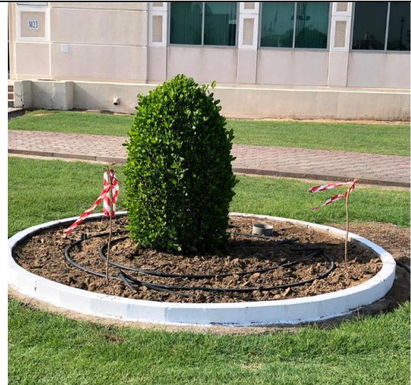
Examples of efficient drip irrigation network (Photo source: University of Sharjah). Plants and flowers in the University are irrigated with a vast drip irrigation system.
