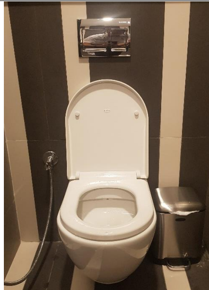
Low flush/dual flush toilets (Photo source: University of Sharjah)
