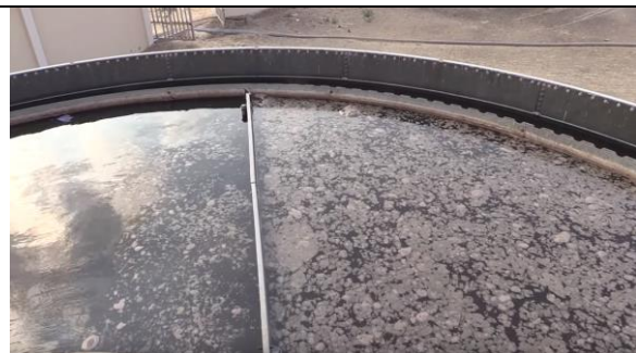
Top Primary (left) and Secondary Right) clarifier of University City Wastewater Treatment Plant
