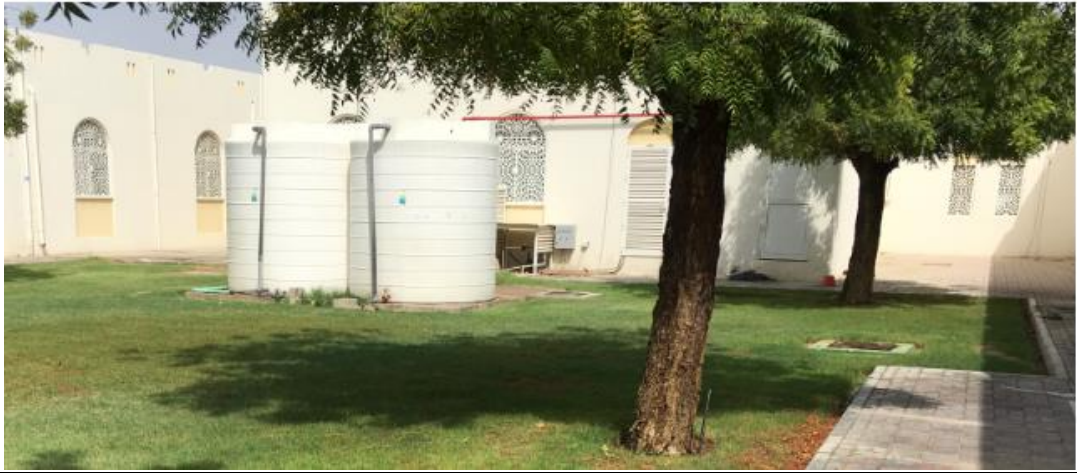
Tanks of greywater recycling system in the student dormitory (Example: University of Sharjah)
