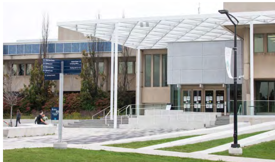
William G. Davis Building expansion
