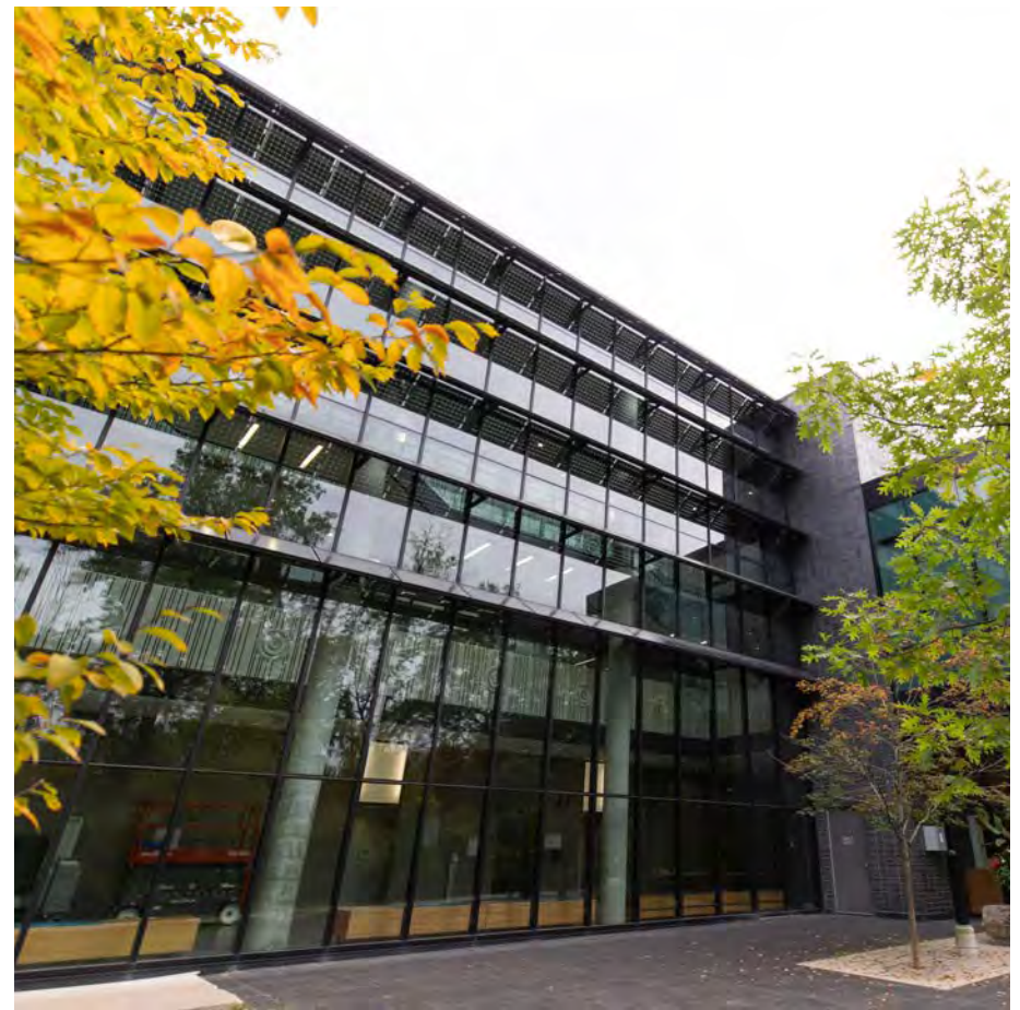
Buildings should consider innovative design to reduce heat gain, such as the brise soleil incorporated into the campus' Instructional Centre.
