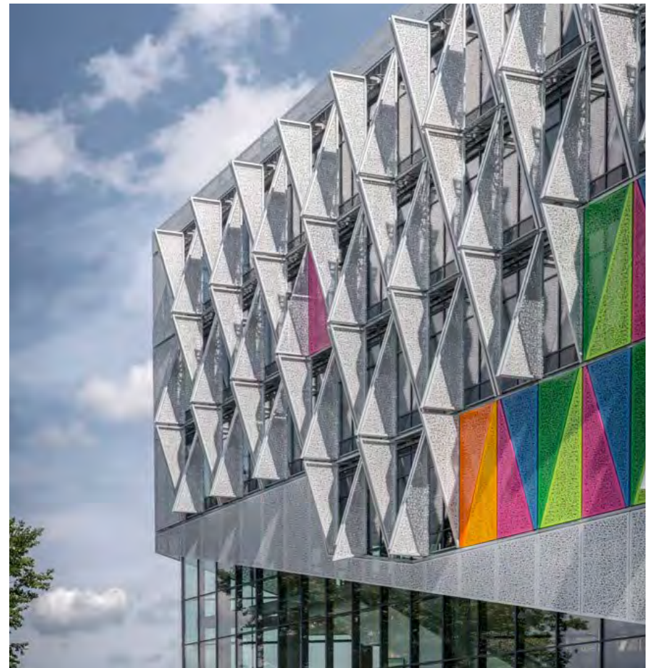
Dynamic solar shading can adjust to climate conditions and user needs.
