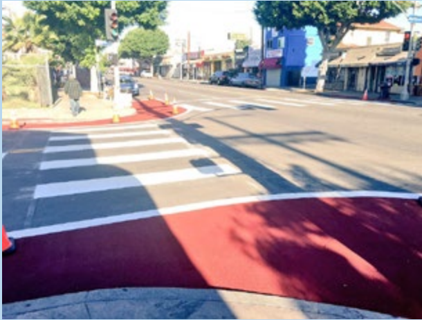
Figure 25: Example of a painted curb extension
