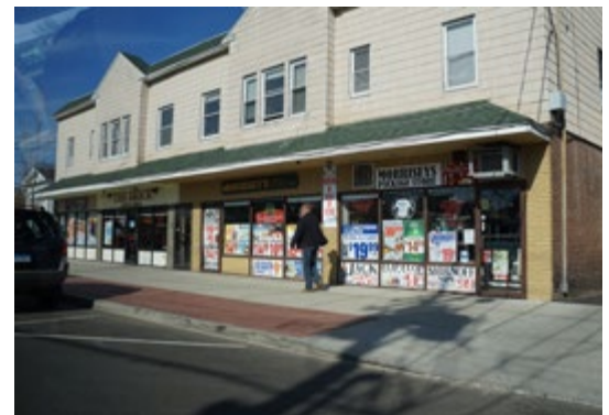
P-D1. The storefront windows and doors on this block of Main Street are cluttered with posters and signs.
