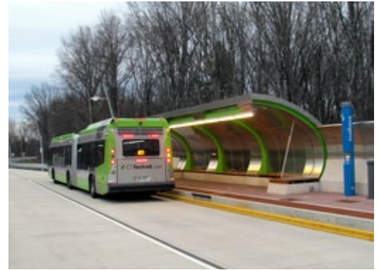
P-R4. Photo of a CTfastrak station
