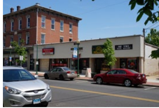
P-D4. Downtown has a variety of building types, architectural styles, ages, and conditions.
