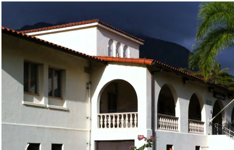
Figure 4.7 Facades: covered arcade and balcony
