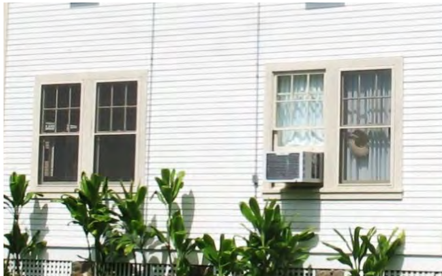
Figure 4.16 Clapboard siding at side elevation
