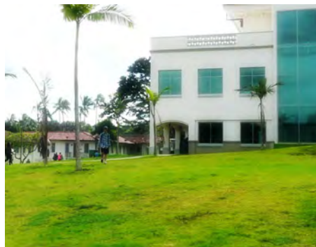
Current condition A
