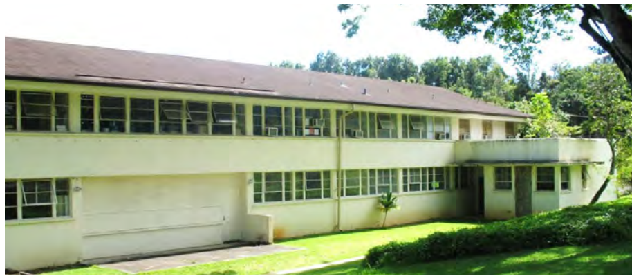
Figure 4.14 2-over-1 steel awning windows
