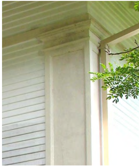
Figure 4.17 Engaged pilaster at exterior corners
