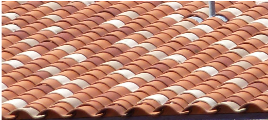
Figure 4.5 Roofs: clay roof tile with multi-color blend
