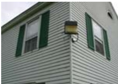
Building-mounted lights provide inconsistent lighting.
