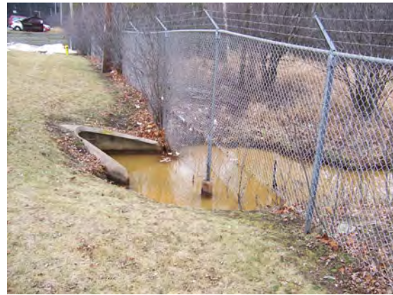
Figure 3-12 – Culvert flowing from the Kmart shopping center (left)
