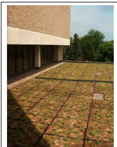
Figure 7-8 - Green Roof Source – UW- Stevens Point
