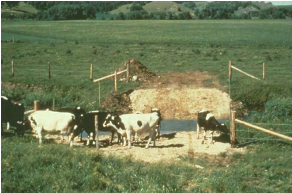
Cattle crossing constructed to minimize streambank erosion and watercourse sedimentation. -photo by Tom Blake
