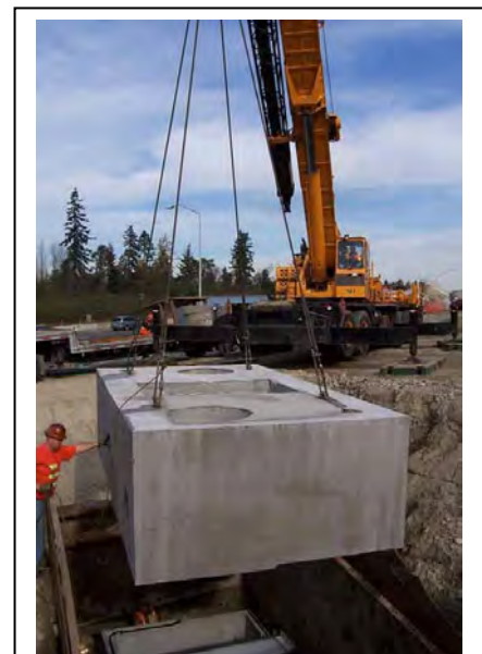
Figure 7-10 - Proprietary Device being installed Source - www.wsdot.wa.gov
