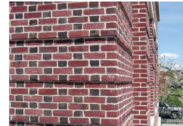
Flemish Bond: Brick, coursed in Flemish bond, may include a two-color scheme for accented areas.
