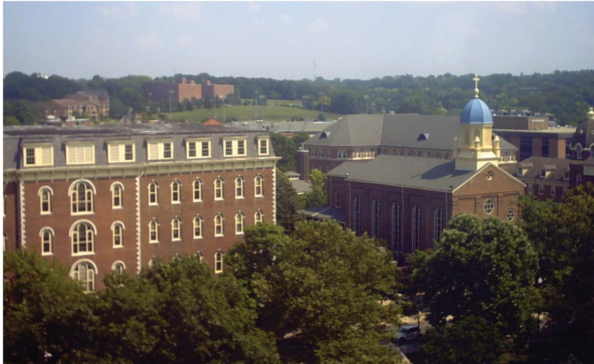
Southeast aerial view of campus; note the various existing roof pitches and massing.
