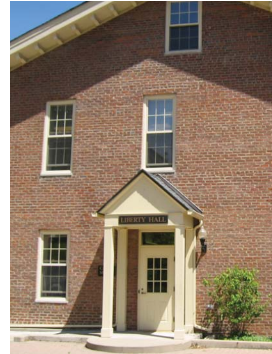
Example of Common Bond at Liberty Hall.
