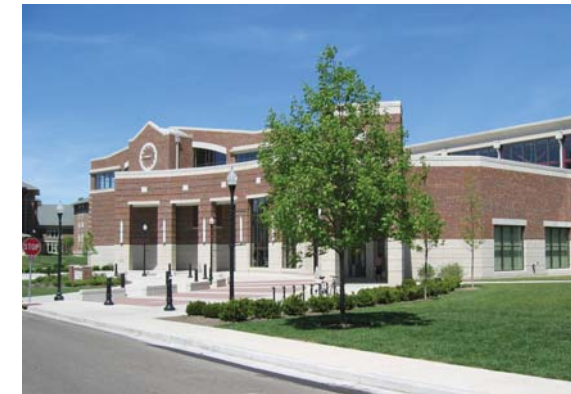
Articulated scale in larger building masses.
