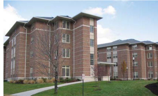
Marianist Hall with a variety of window types set in a common rhythm on the façade
