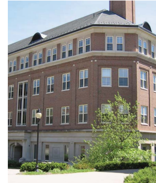
Running Bond is used at the Humanities Center, with limited areas of soldier coursing and special shapes for additional detail.
