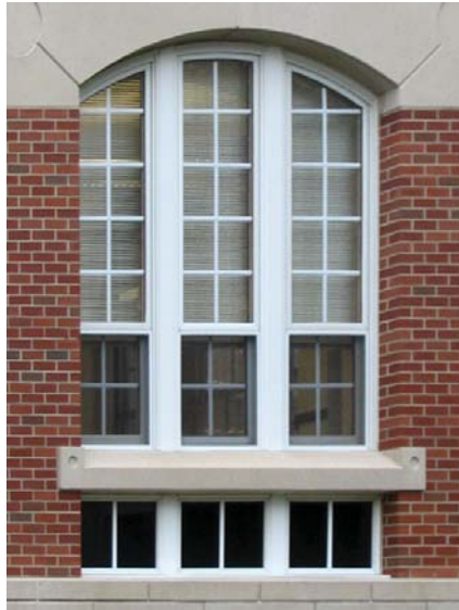
Divided lights are encouraged for their contextual relationship to other campus buildings, and to humanize the scale, as in this example of Keller Hall.
