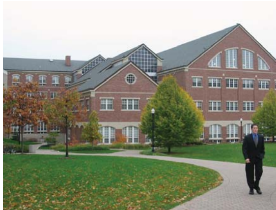
Fixed window wall assemblies in the rear gable of Keller Hall support and announce the interior function of the space behind them.
