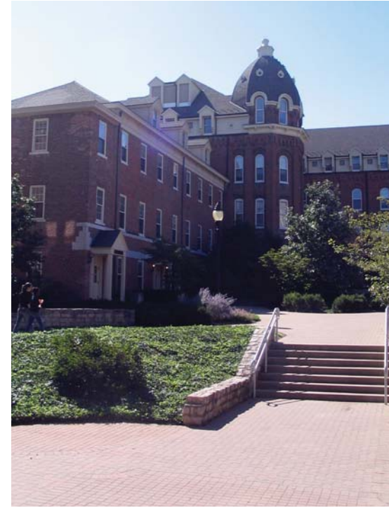
Elevation changes along the path act as thresholds and help denote separations of space within the campus network.
