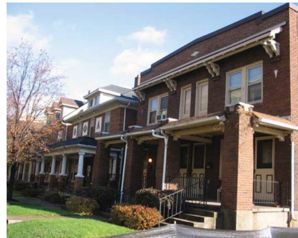
Existing student neighborhood housing in brick
