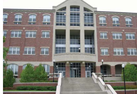
Double-hung windows are the preferred operable type, organized in individual, paired, and triple units as in Keller Hall.
