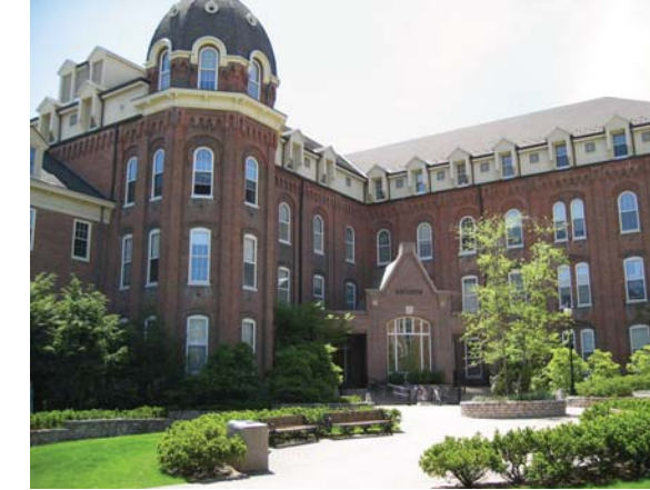
The Nazareth Courtyard entrance to St. Joseph Hall uses a projected addition, reaching out into the prominent corner of the courtyard. The entrance addition is not the dominant element of the building façade, but still serves as the entrance beacon. Its gabled form is contextual with St. Joseph Hall, and its scale is reduced to the pedestrian level, becoming a part of the courtyard as much as the building.
