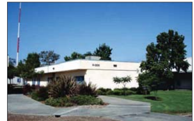
K-300: Computer Labs, Classrooms
