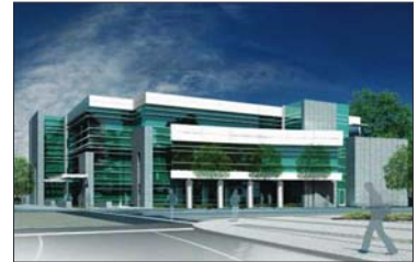
New Allied Health Building - Under Construction
