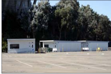
T1, T11, T3: Temporary Classrooms
