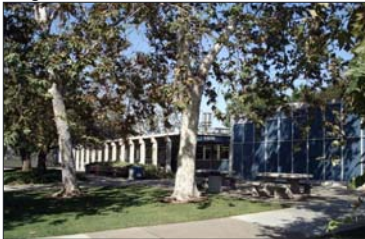
I-100, I-100: Classrooms
