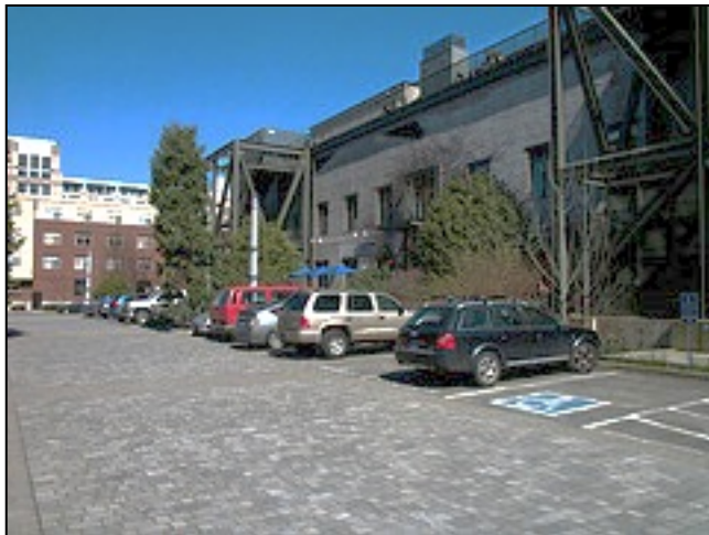
Figure 38 Permeable paver parking lot.
