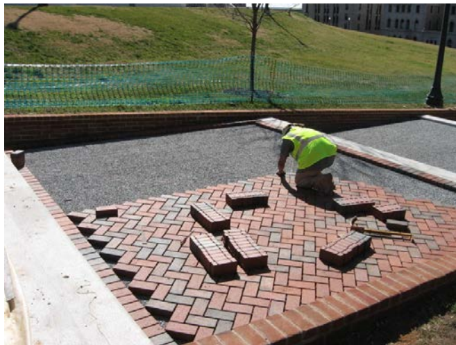
Figure 32 : Permeable pavement system
