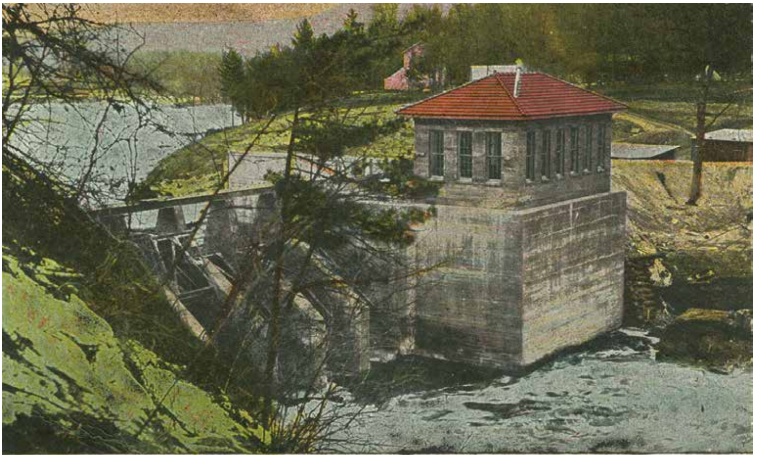
189.—Concrete Dam, Upper Iowa Power Co., between Decorah and Waukon, Iowa.
