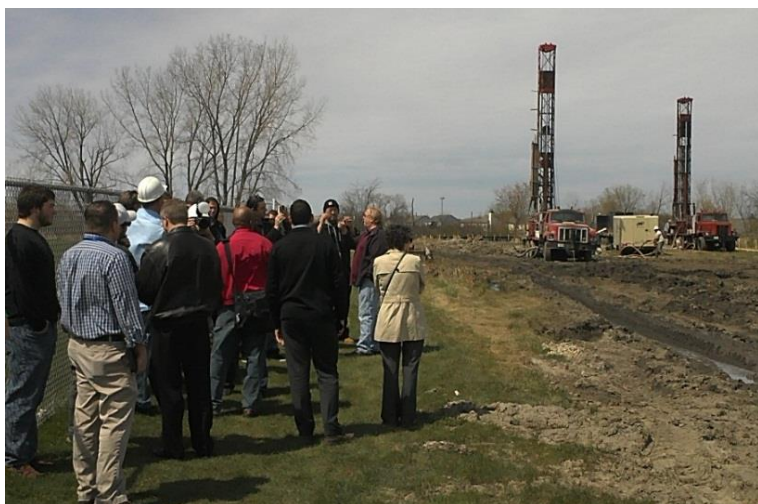
CLC HVAC students meeting with geothermal well drill team
