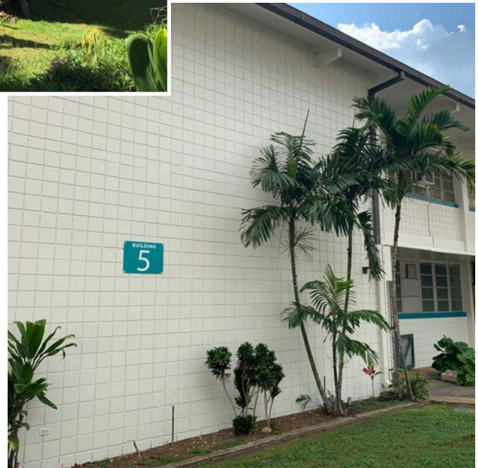
Building 5 Renovations Expected Completion Date: April 2021
