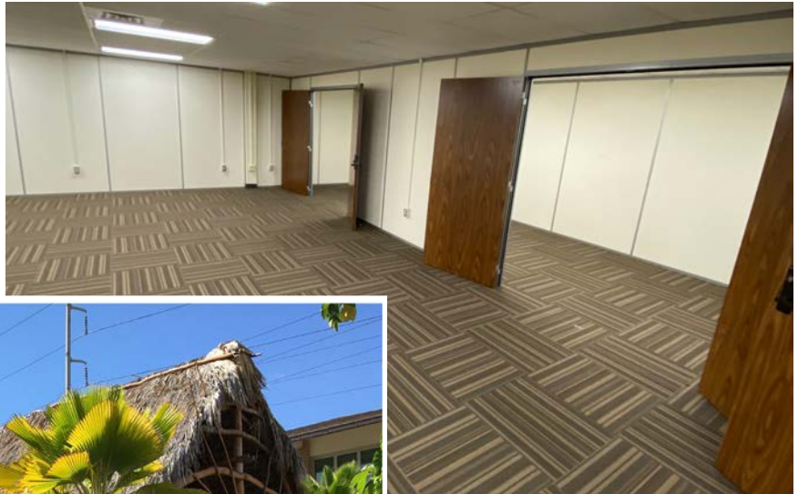
Building 72A Expected Completion Date: February 2021
